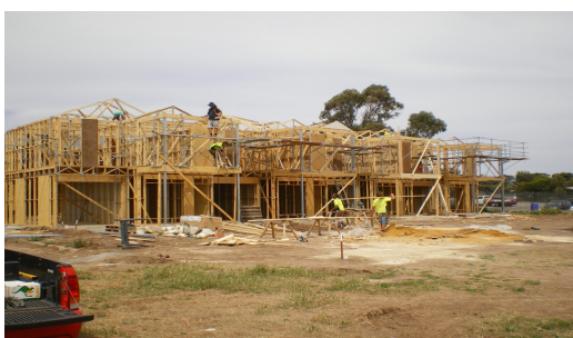
Anniversary Apartments Project under construction 2010
